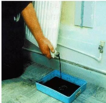
Accumulation of sludge is an indication of corrosion in the heating system and may also be accompanied by the accumulation of gases within the radiators – which may be mistaken for air when a radiator is bled.
